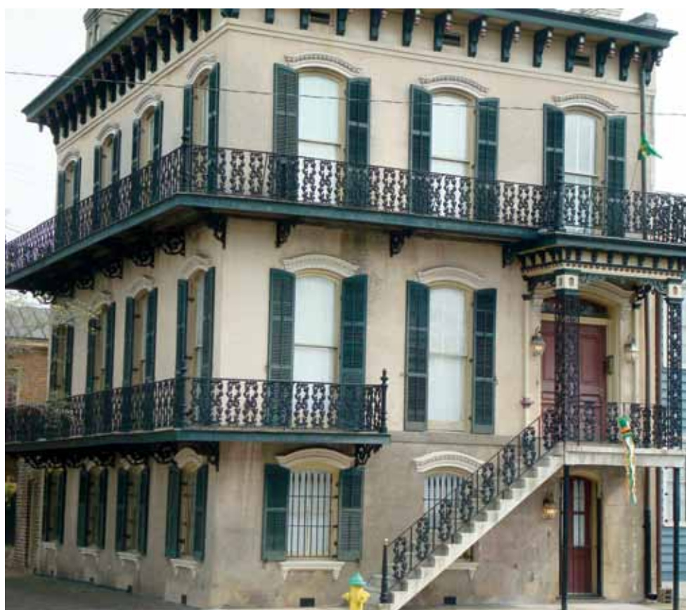
This looks like it could be a classic example of New Orleans' French Quarter architecture but this one of many historic homes we saw in Savannah.
